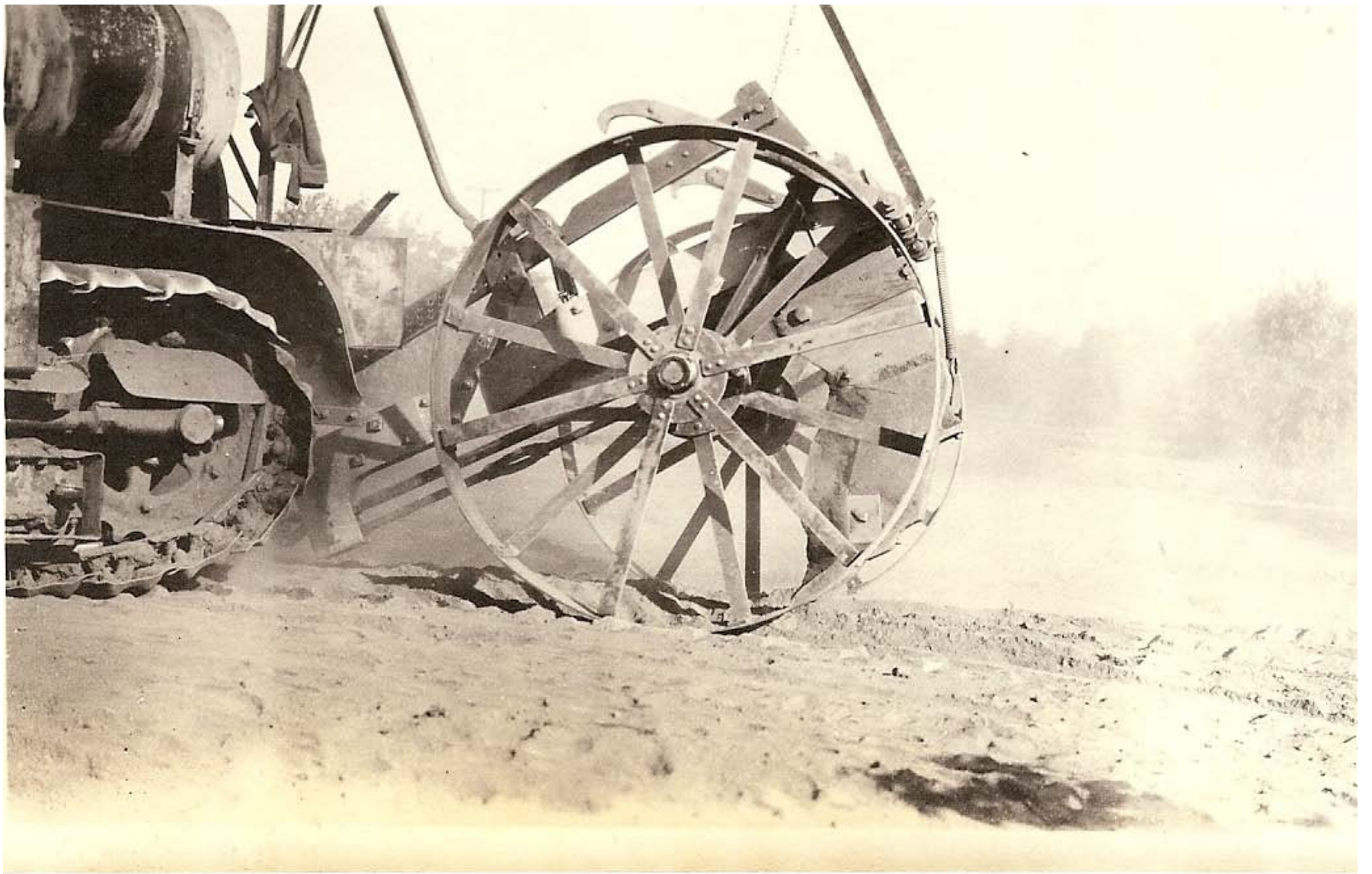
Soil ripper. Source: Alan George, Norm Phillips and Wayne Collins.
