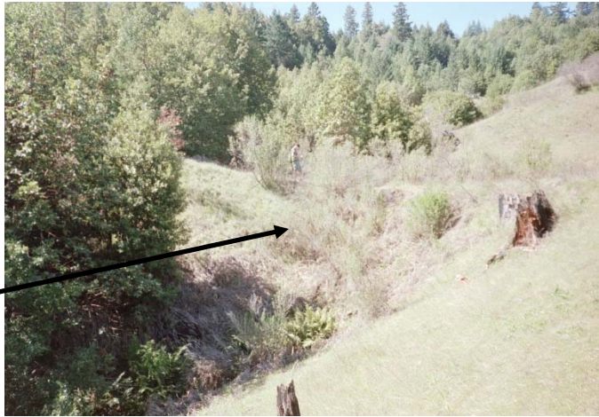
Example Road Related Diversion Gully (8 meter width, 8-10 meter depth)
