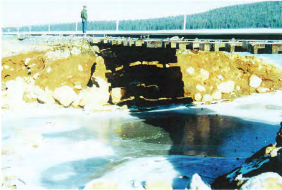
Figure 12. Union Pacific Railroad grade washout in the vicinity of County Rd 112 and Highway 44. January 1997.
