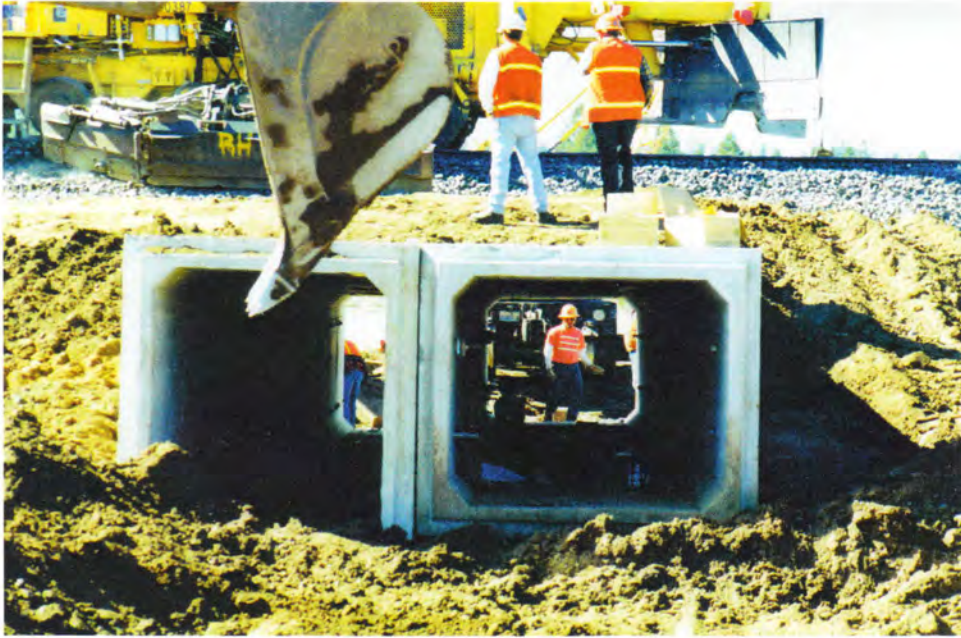
Figure 18. Concrete box culverts under BNRR line near Highway 44. Note left culvert installed on side and below grade to create fish passage channel.
