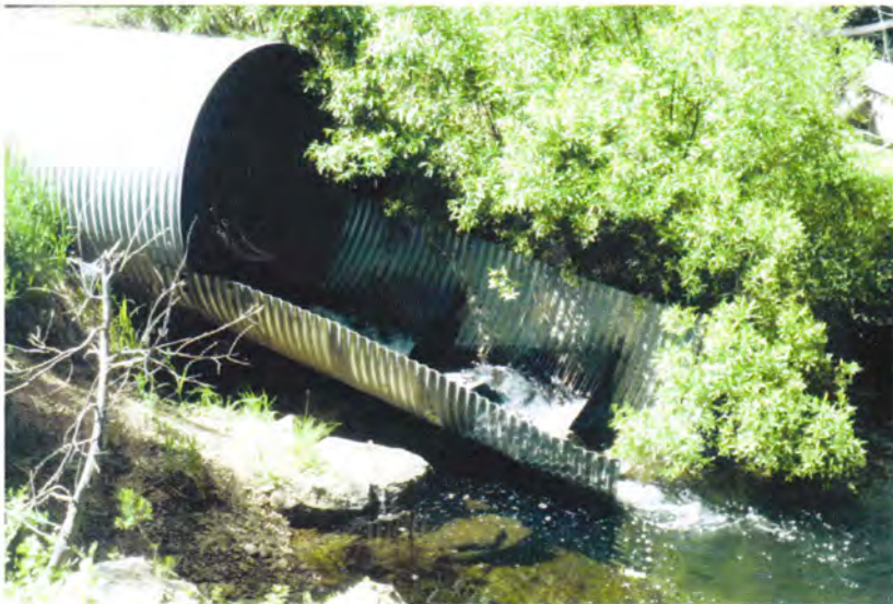
Figure 16. Top, Pine Creek looking downstream after removal of culvert and road crossing, 10/1997. Bottom photo showing baffles on lower end of culvert in an attempt to provide for fish passage 1978.
