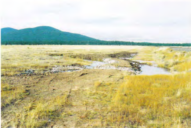
Figure 19. Berms constructed and/or repaired in 2005 to prevent or reduce flows into borrow ditches alongside BNRR grade in Pine Creek Valley.
