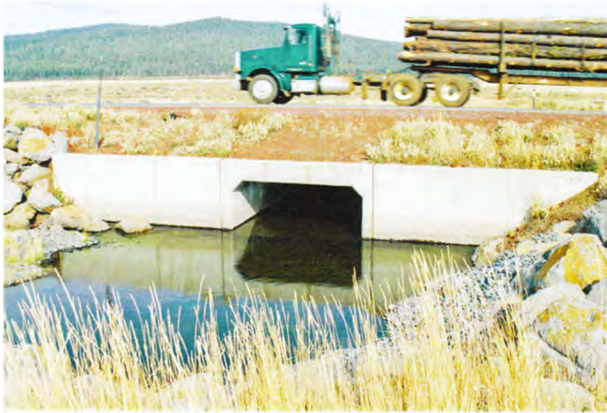
Figure 17. Culvert under Highway 44 on mainstem of Pine Creek, upstream side. 11/05.
