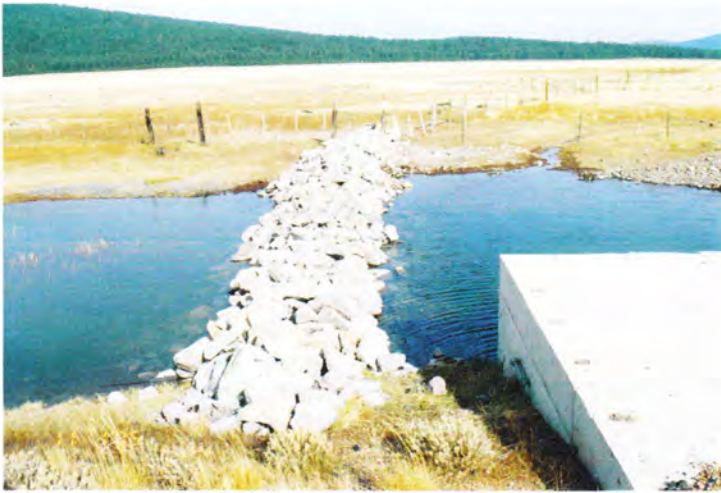
Figure 18. Concrete box culverts under BNRR line near Highway 44. Note left culvert installed on side and below grade to create fish passage channel.
