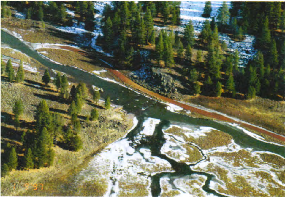
Figure 27. Above, Bradford three-step rock structure constructed in 1995. Bottom, aerial view showing stream backed up into the valley.
