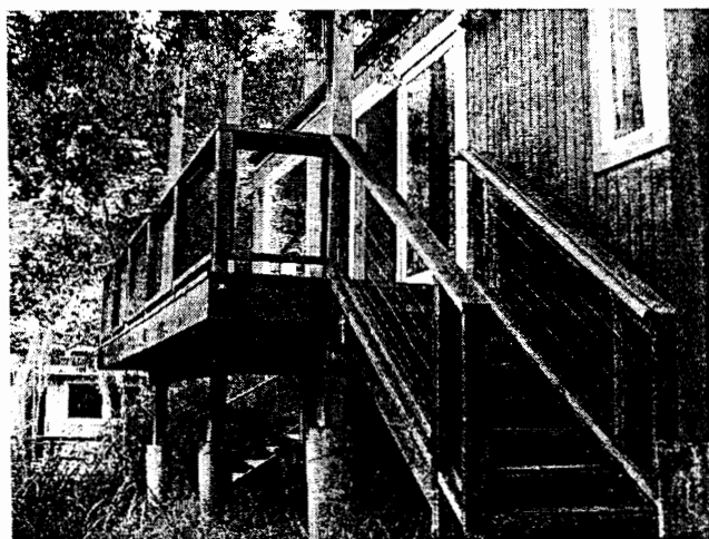
Figure 1. ~ In the UWI, attached decks would be subjected to under-deck flame-impingement exposures and above-deck burning brand exposures.
