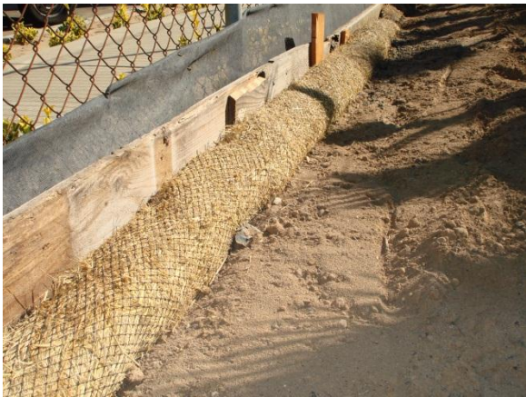
Straw wattles absorb runoff and sediment.
