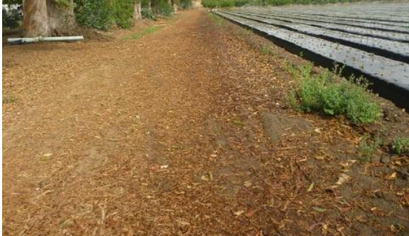
Mulched or seeded roads reduce sediment movement and may increase water infiltration.
