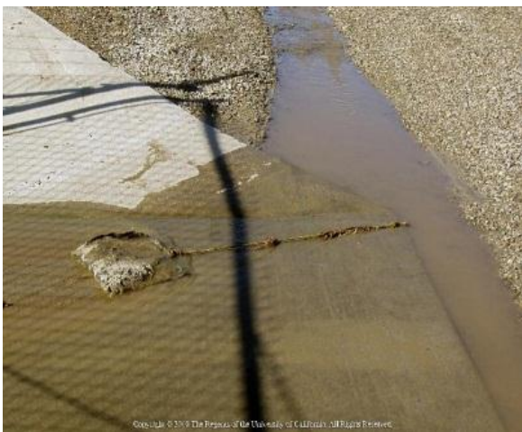
Polyacrylamide in an anchored bag binds to sediment in a runoff capture area.
