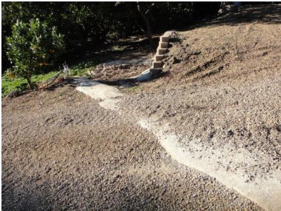
A waterbreak reduces flow down the full length of a road.
