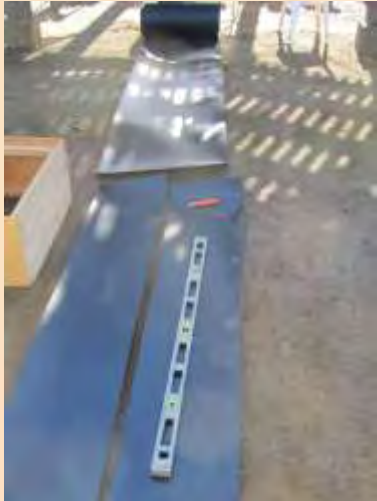
Cutting 30-inch wide bamboo barrier in half; 15-inch used for beds
