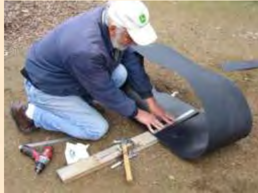
Connecting the ends
