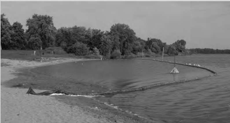
Figure 8.2 Enclosed bathing area and intake for on-shore UV system at Fanshawe Beach, Ontario, Canada.
