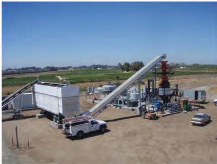
Figure 3 – A P500 installation in California
