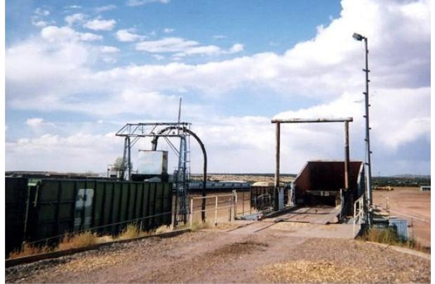
Truck-to-rail reload showing the truck dump, Fort Apache Timber Company, Snowflake, AZ. Source: USDA Forest Service
