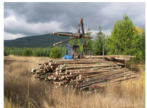
Small-scale forwarder unloading smallwood pulp and hog fuel "logs" from overgrown Christmas tree plantation thinning operation in Bonners Ferry, Idaho. October 2008. Photo by Barry Wynsma, USFS
