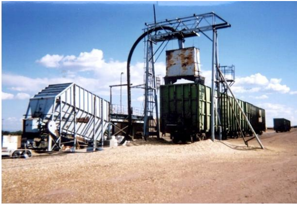
Truck-to-rail wood chip reload facility. Fort Apache Timber Company, Snowflake, AZ. Source: USDA Forest Service
