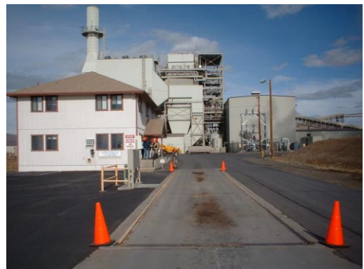
Weight scale and Scalemaster's shack at HL Power's 35 MW power plant in Wendel, California. November 12, 2002. John Stewart
