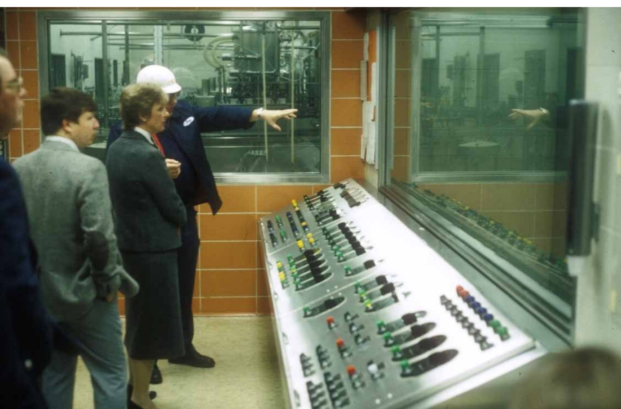
Control Room at Safeway Processing Plant
