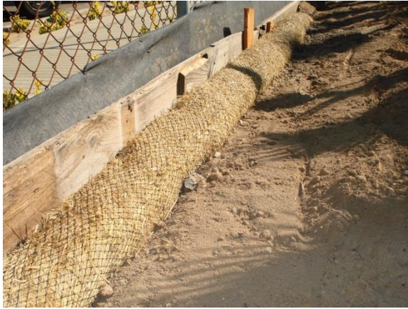
Straw wattles absorb runoff and sediment.
