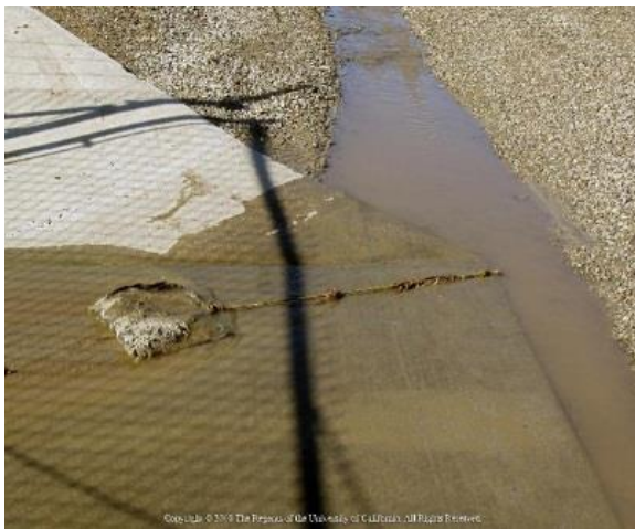
Polyacrylamide in an anchored bag binds to sediment in a runoff capture area.
