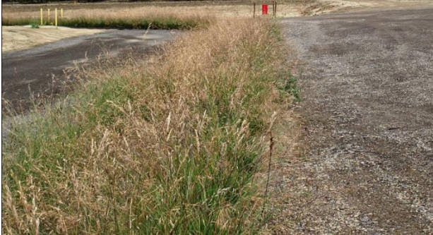
Vegetation along the road minimizes off-site movement of runoff and sediment.
