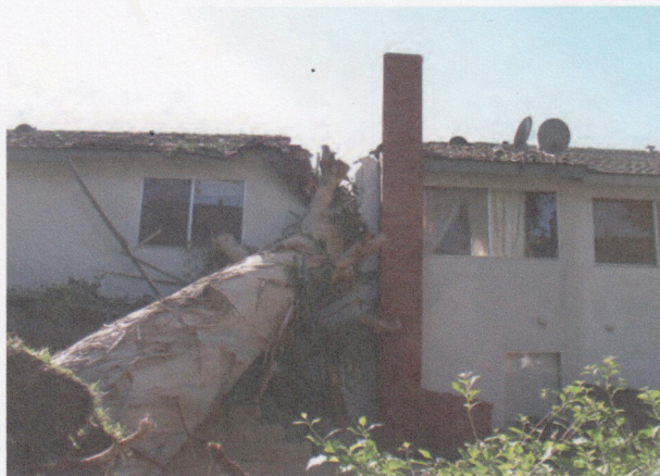
Figure 1. Property damage is not uncommon when trees fail. Here, a large blue gum caused considerable damage to this house. Photo: T. Larson
