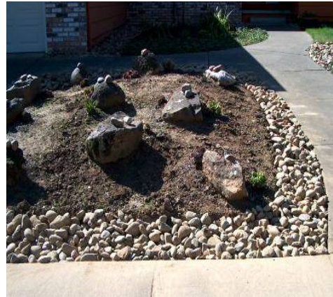
1/3 of trench filled with gravel and topped with cobbles.
