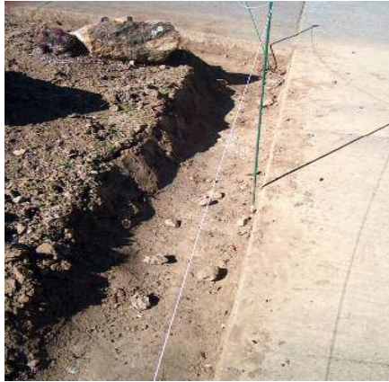
1'x2' trench dug around 12'x15' area
