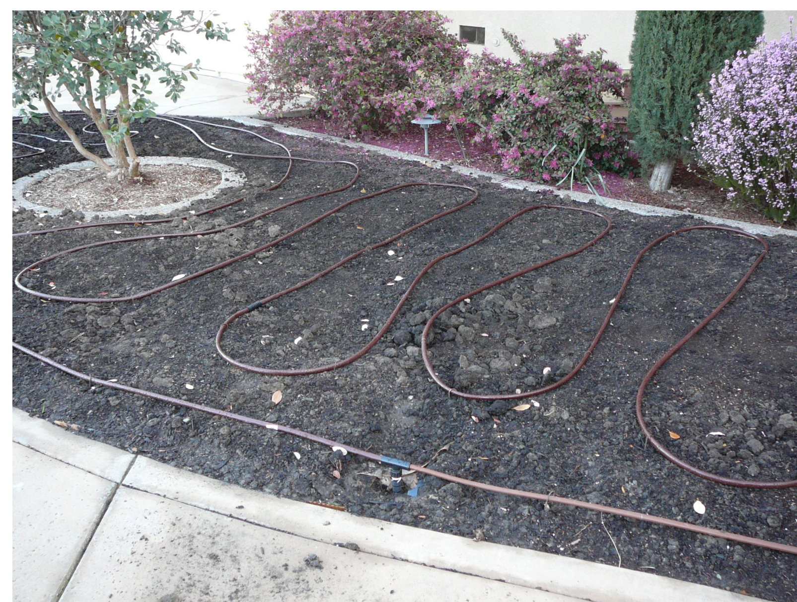
Exhibit D: Irrigation placement of Netafim™ or other drip-type irrigation on the topsoil.
