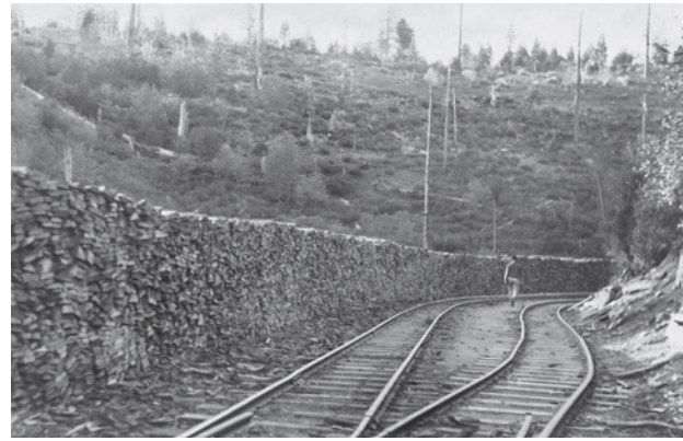
FIGURE 36.2 Logging railroad of the Michigan–California Lumber Company close to Pino Grande, El Dorado County, California, showing piles of slab wood fuel for the railroad engines, May 1925. Though slab wood was an expensive form of fuel, its use meant closer utilization of the forest products. Photo: Courtesy of the Marian Koshland Bioscience and Natural Resources Library, UC Berkeley < http://lib.berkeley.edu/BIOS >.
