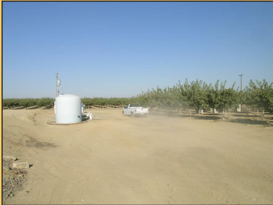
Poles in tree rows are susceptible to topping.
