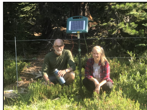
Temporary fencing was installed with assistance from the Feather River Land Trust to exclude livestock until fen vegetation can re-establish
