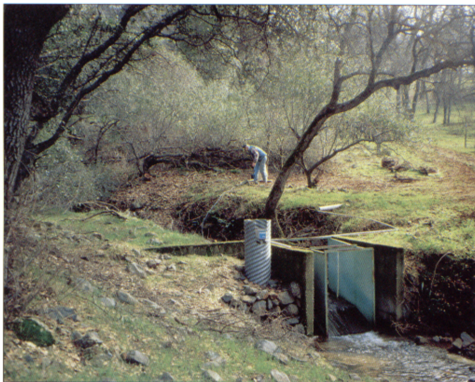
Stream flow is measured and recorded every 15 minutes.
