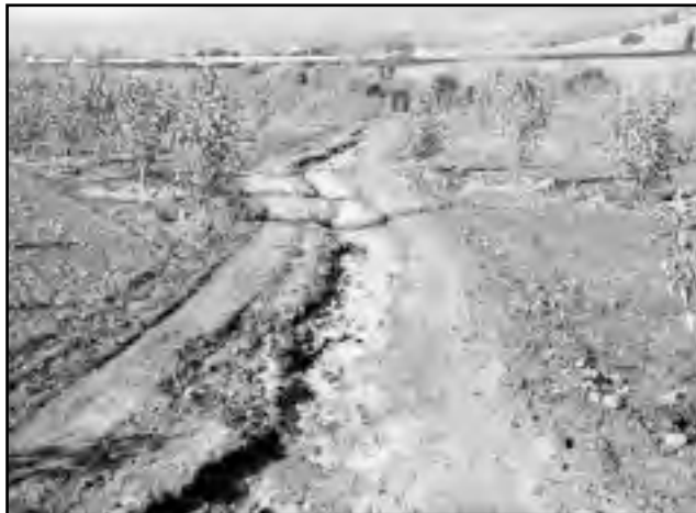
Erosion ditch before revegetation.
