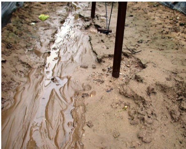
Erosion path from tunnel runoff
