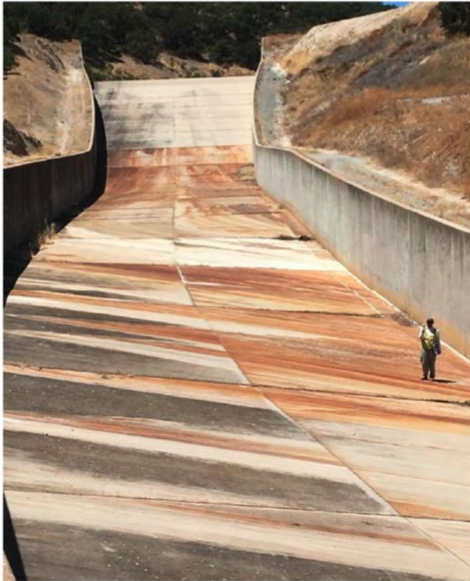
Upstream Portion Spillway Chute
