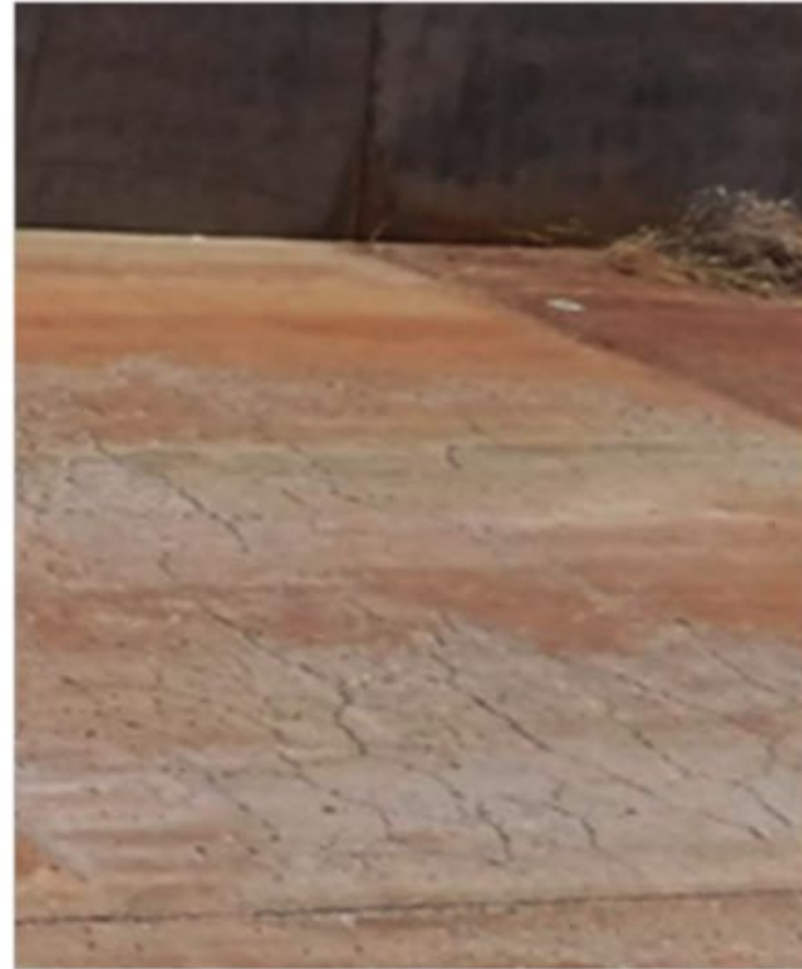
Example Concrete Condition
