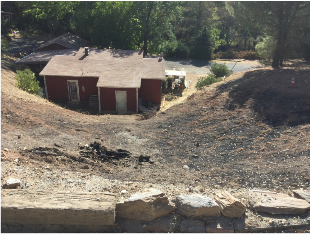
Residence in the drainage path of a small basin tributary to Murray Creek. The upstream side of the culvert is approximately half filled with sediment, the downstream side is buried in artificial fill. The basin upstream of the culvert experienced moderate-to-high soil burn severity.
