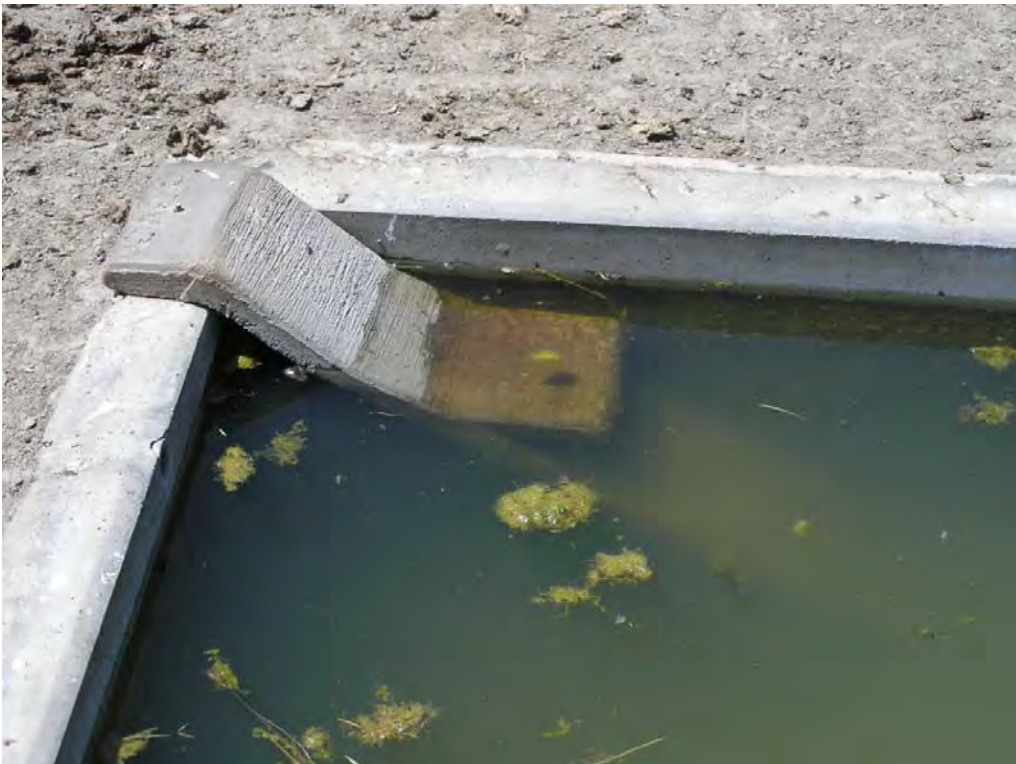
Figure J-1. Example Watering Facilities with Hardened Surface and Wildlife Escape Ramp
