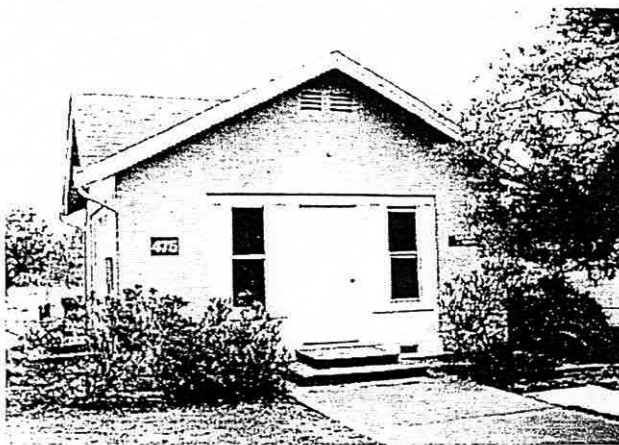
Figure 6. ~ The woodframe structure (Villa Termiti) built specifically as a test bed for efficacy trials involving detection devices, non-chemical and least-toxic management methods.
