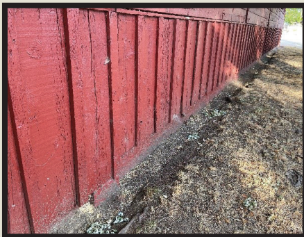
Barn with combustible wood siding has low susceptibility to surface fire with litter and vegetation removed.
