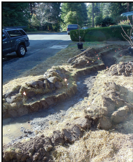
The long stream bed keeps water flow rates down, letting it infiltrate the soil.
