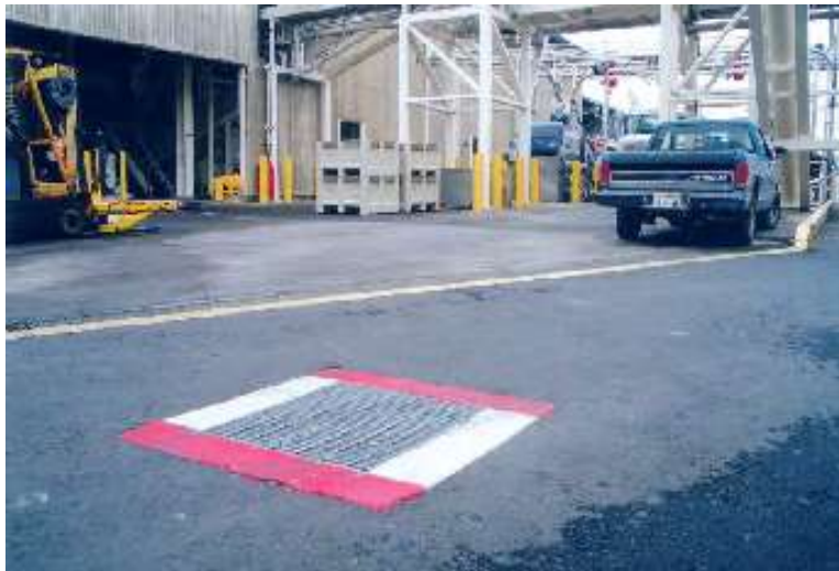
Clearly marking storm drains helps to keep them clear of hazardous materials and waste.
