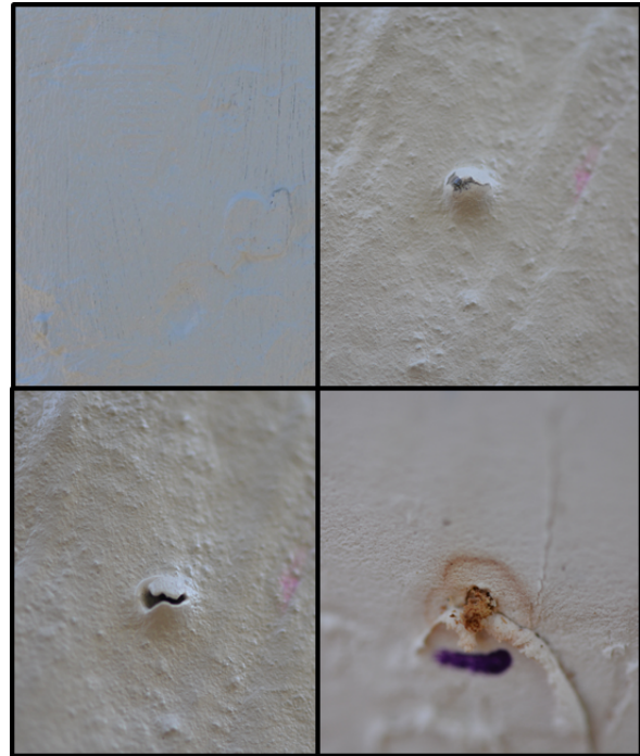
Figure 4: Progression of beetle reemergence after paint application. After paint application has begun to dry (A), the female beetle will begin to re-establish the entry point with her abdomen (B), break through the paint obstruction (C), and continue to maintain the gallery (D).
