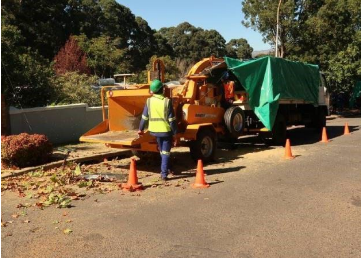
Trees are chipped on site. (City of Cape Town)
