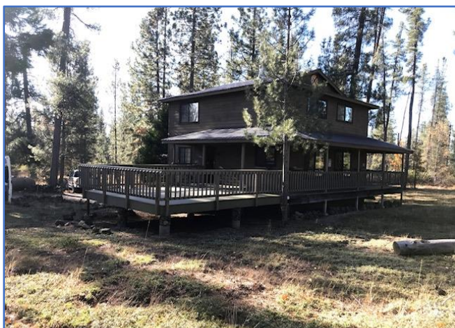
Figure 3. Defensible space and tree removal completed by workshop participant, Lassen County May 2022.
