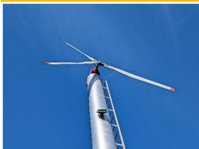
This three-bladed propeller is notably quieter than industry-standard two-bladed propellers, but provides slightly reduced coverage. In areas where neighbor noise impacts are problematic this can be part of the solution.
